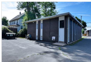
New roof, fresh paint, new floors - the hard work is already done
